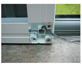
**To alter the width of the Folding Flyscreen** cut the top and bottom profiles to the required width. Always allow for the corners which measure 4cm each. (NOTE the 4M width of the folding material cannot be reduced).
