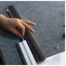
Cut the metal profiles 4cm less than the required height to allow for the corners. Cut the mesh screen 3cm less than the required height.
