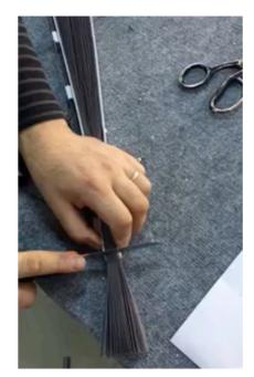
Cut the white plastic backing on the mesh screen with scissors by 0.5cm on both sides so that it will sit in the corners correctly.
